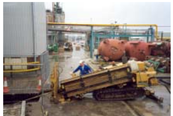
Drilling within the plant
